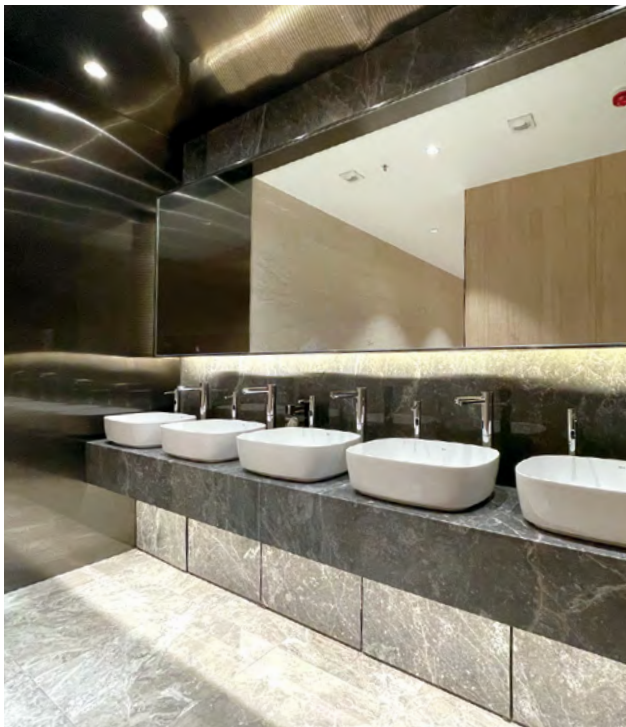
亞博館內的洗手設施及廚房均安裝 Ozone 淨水消毒系統，務求加強公眾對館內衛生安全的信心 The Ozone Water Disinfection System has been installed in washrooms and the central kitchen at AWE to enhance public confidence in its hygiene
