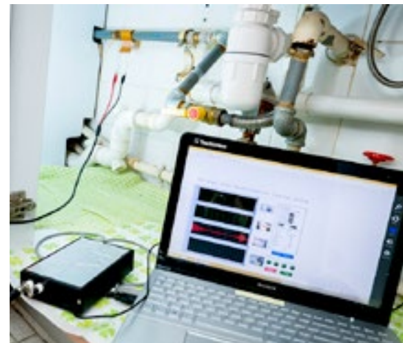
上圖顯示利用城大系統檢測住宅廚房的煤氣喉管；左邊的長方型小盒為 USB 數據收集裝置。 The system developed by CityU team is shown here examining a gas pipe in the kitchen of a flat. The small box on the left is a USB-based data acquisition box.
