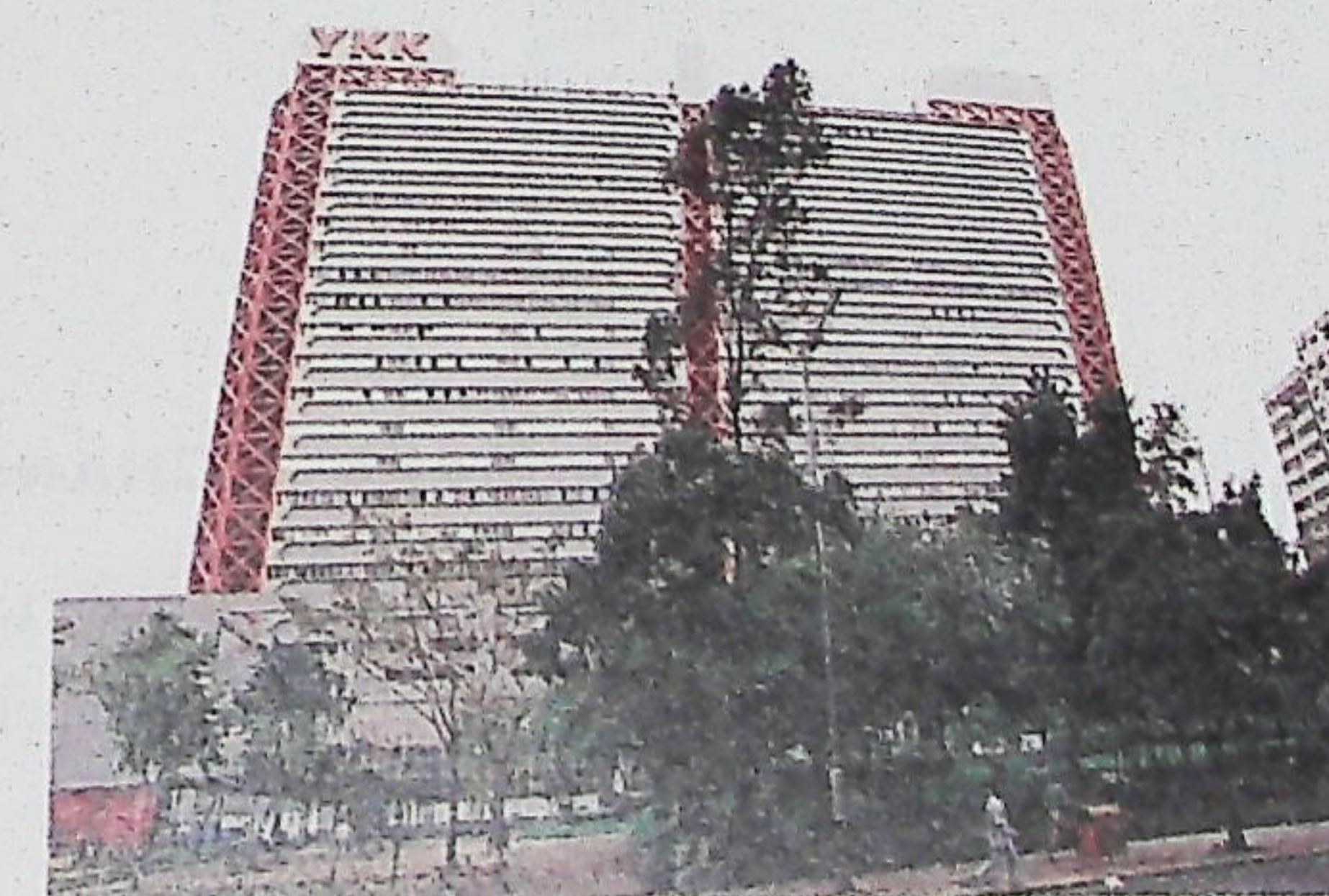
A new industrial building in Tuen Mun.
