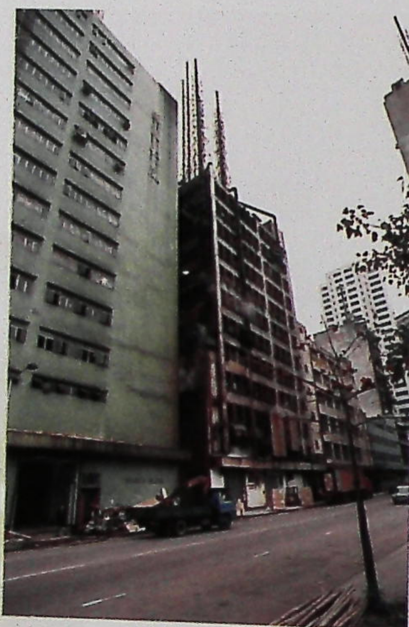
Old industrial buildings.
