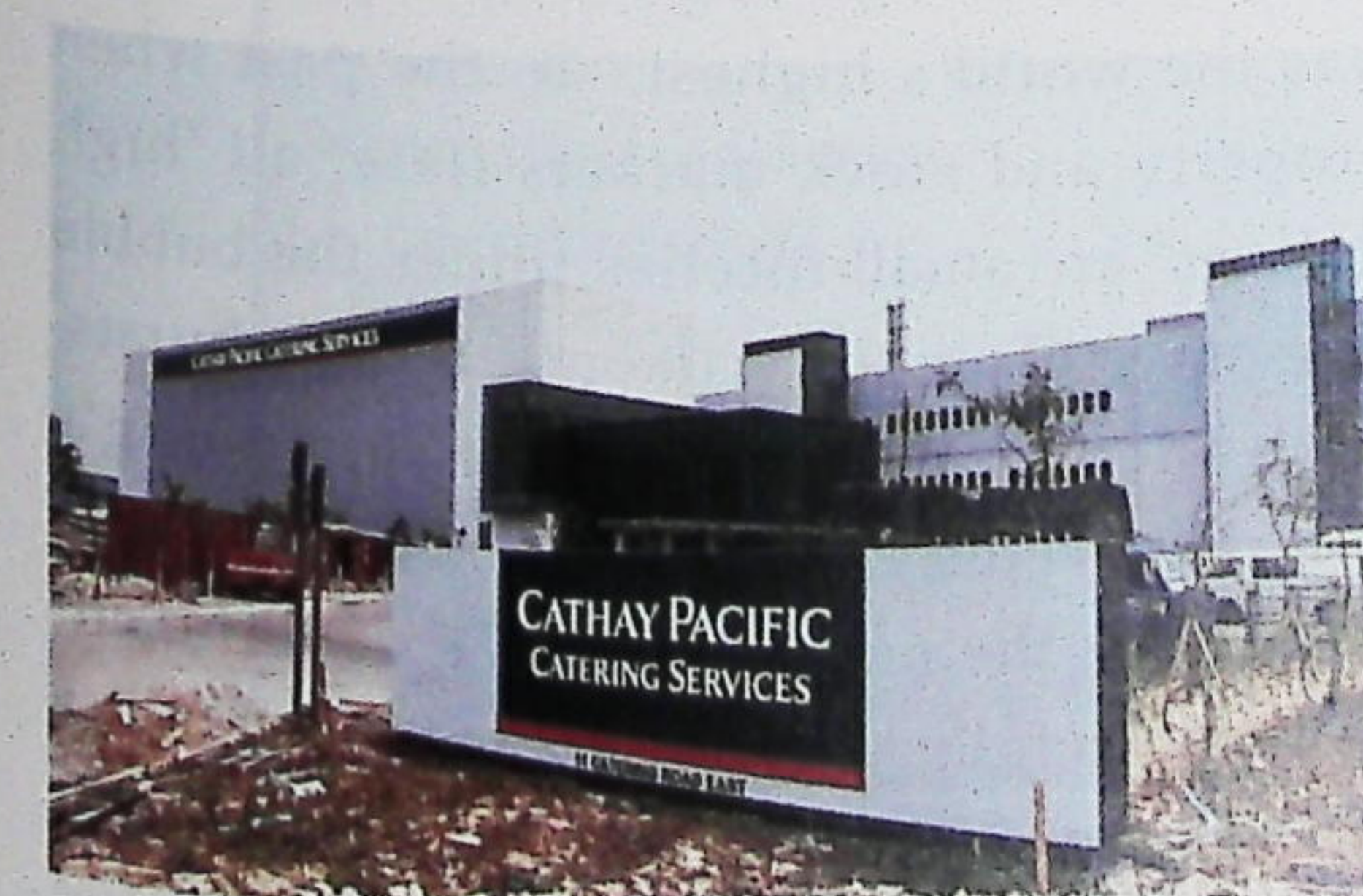
The new inflight kitchen has a maximum capacity of 80,000 meals per day.
