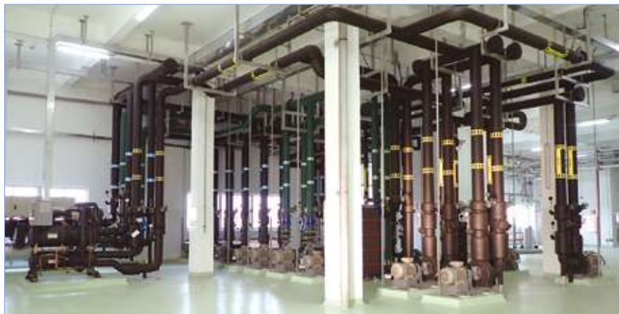
地源磁懸浮冷水系統是李錦記獲得2025年香港ESG獎的「ESG大獎」的核心項目 The ESG Grand Award was presented to Lee Kum Kee in recognition of its groundbreaking geothermal magnetic suspension chiller system
